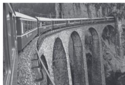
Landwasser Viaduct, Switzerland
